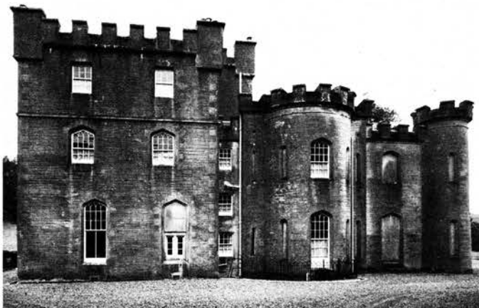
View of east side of house showing the tower-block which was added to the original house.
