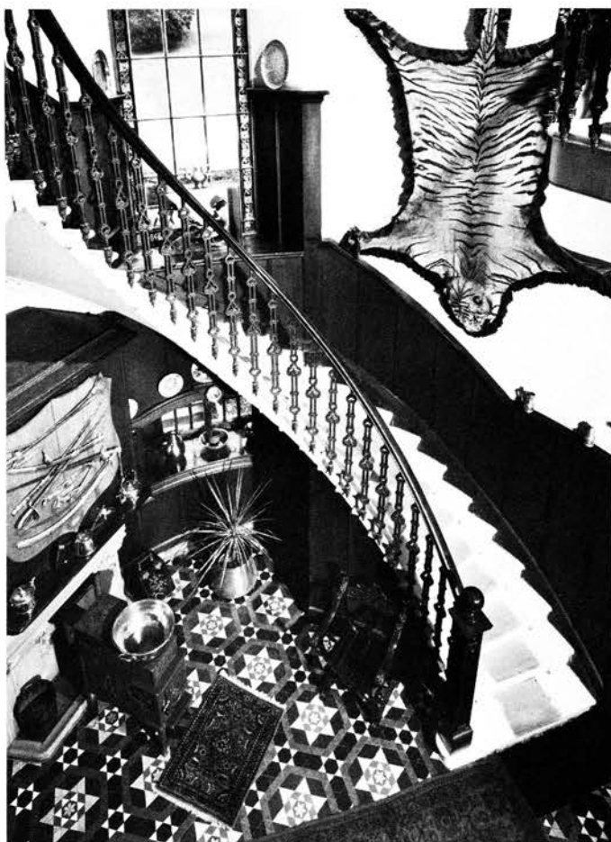
Gallanoch's cantilevered stair which was installed when the entire rear portion of Burn's design was omitted. (By permission of the Royal Commission on the Ancient and Historical Monuments of Scotland.)
